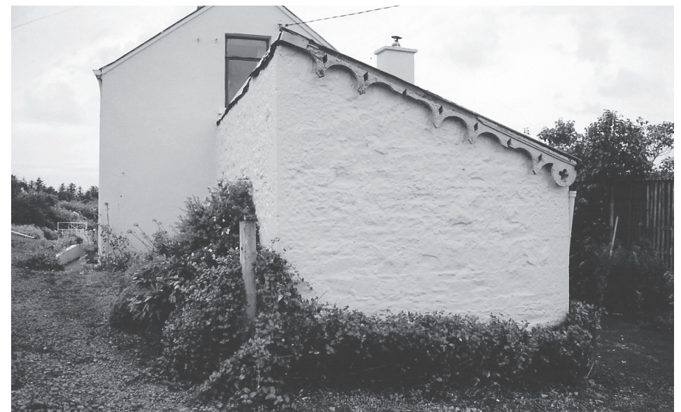
Former Drumemin Station
